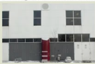
Existing Steel Construction
